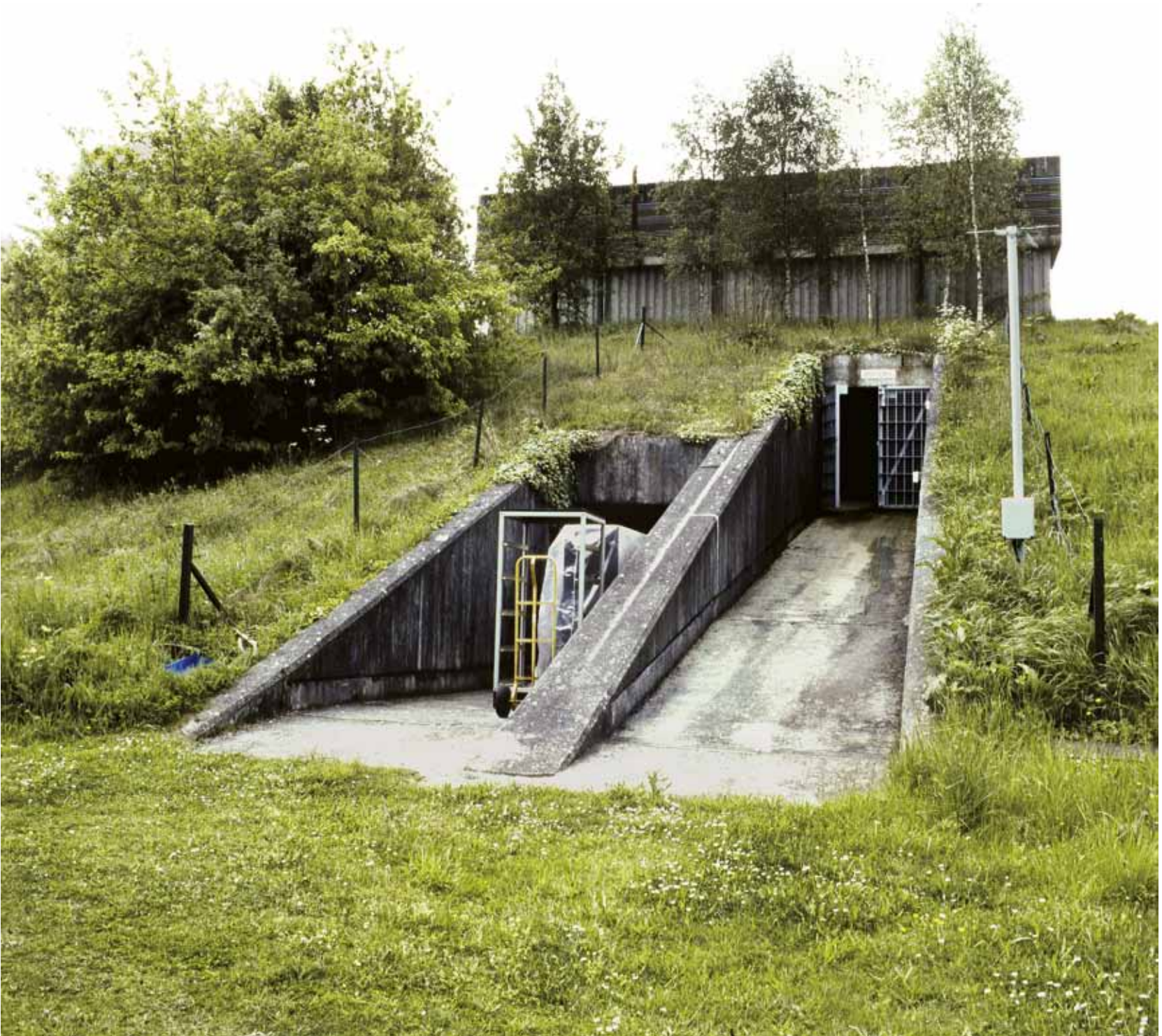
Above: The principal entrance to the bunker, with the ventilation towers on the hillside above. The left-hand incline gives access to the service areas on the lower level, including the generators and air-conditioning plant. The right-hand incline accesses the main administrative areas of the bunker. Both entrance portals give onto narrow, dog-leg corridors terminating in massive steel blast doors that secure the main body of the bunker.
