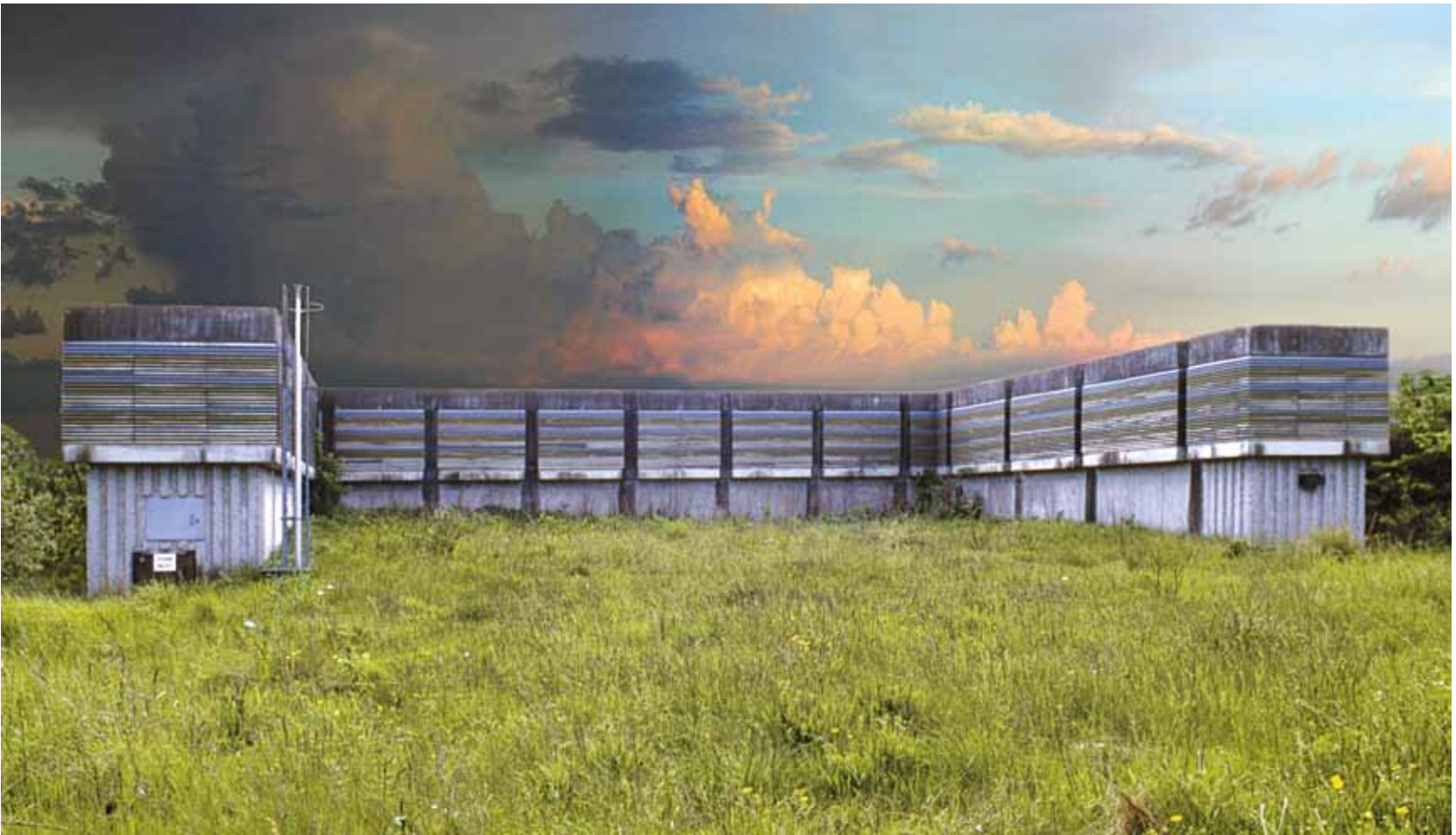
Above: The somewhat sinister outline of the Chilmark ventilation towers provides a surreal backdrop to the valley of the river Nadder in Wiltshire.
